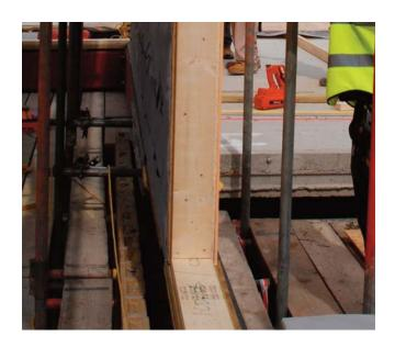
Racking resistance of a SIP wall is typically 50% greater than that of a timber studwork wall sheathed with one layer of 9mm OSB. Therefore a low rise building designed to be constructed with loadbearing timber studwork, should also work with a loadbearing SIP structure. A structural engineer would need to confirm this by calculation.
