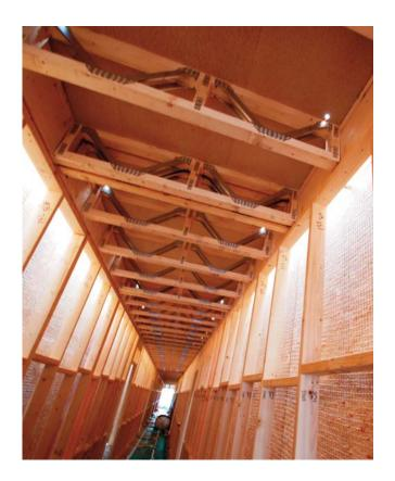
These types of wall, although lightweight in their nature, are actually capable of outperforming many masonry party walls. Onsite testing has shown that these types of wall generally achieve airborne sound insulation test results some 10 dB better than Building Regulations minimum standards.
