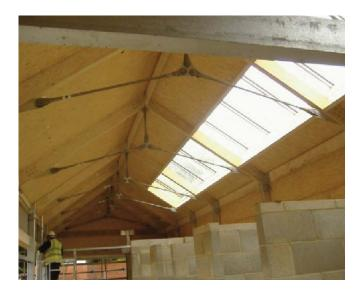
Coverings for pitched SIP roofs can be any type of covering that may be used on any other type of roof (e.g. tiles, slates, profiled metal etc). A ventilation void must be provided between the SIP and the roof covering, so the use of counter battens before tiling battens, profiled metal roofing or any other covering should be considered. Roofing battens should be fixed to the SIP roof with the use of screws.
