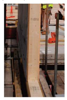
loads. Whilst this is not impossible, it does present practical and economic limitations. SIPs used as infill panels is a practical and economic way of adding thermal insulation and infill structure to steel or concrete frame buildings, and allows a rapid cladding of the structural core with large panels craned into position.
